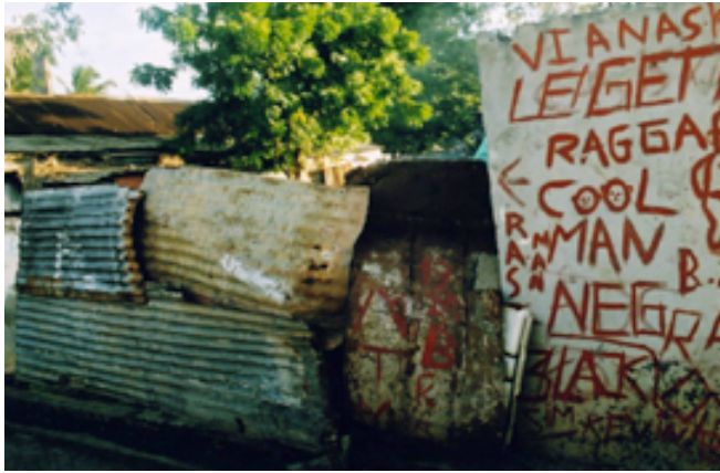
Chagossian housing in Cassis: most of the homes are built of corrugated iron, which rusts in the wet
