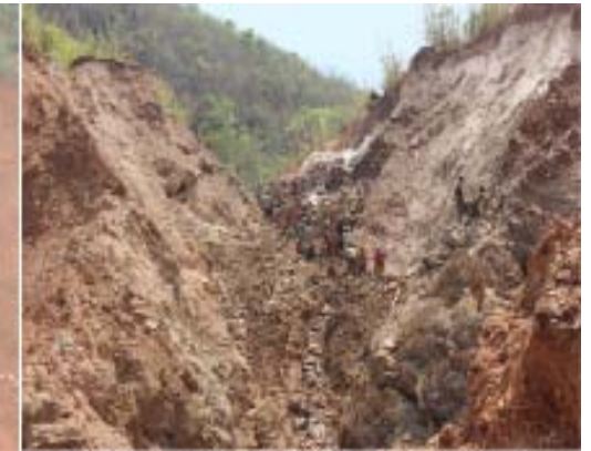
Landslide on 25 April, 2012
