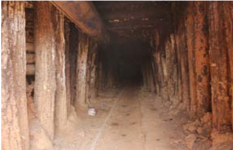
Logs are used to prop up the roof in one of the Mawchi mine tunnels
