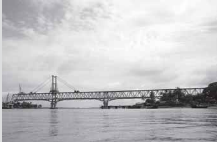
The bridge while under construction
