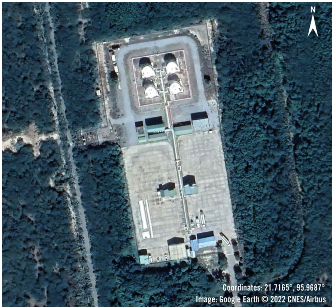
NEPAS storage facility at Mandalay airport.
