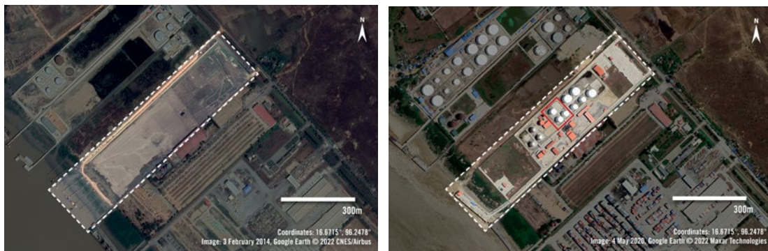
Puma Energy Terminal, Thilawa, Myanmar: Satellite imagery shows the Puma Energy Terminal while it was under construction at Thilawa (2014) and later in 2020, when the terminal appears to be operational. According to a company video, the three tanks used for jet fuel storage are shown in the image – highlighted with a red square.
