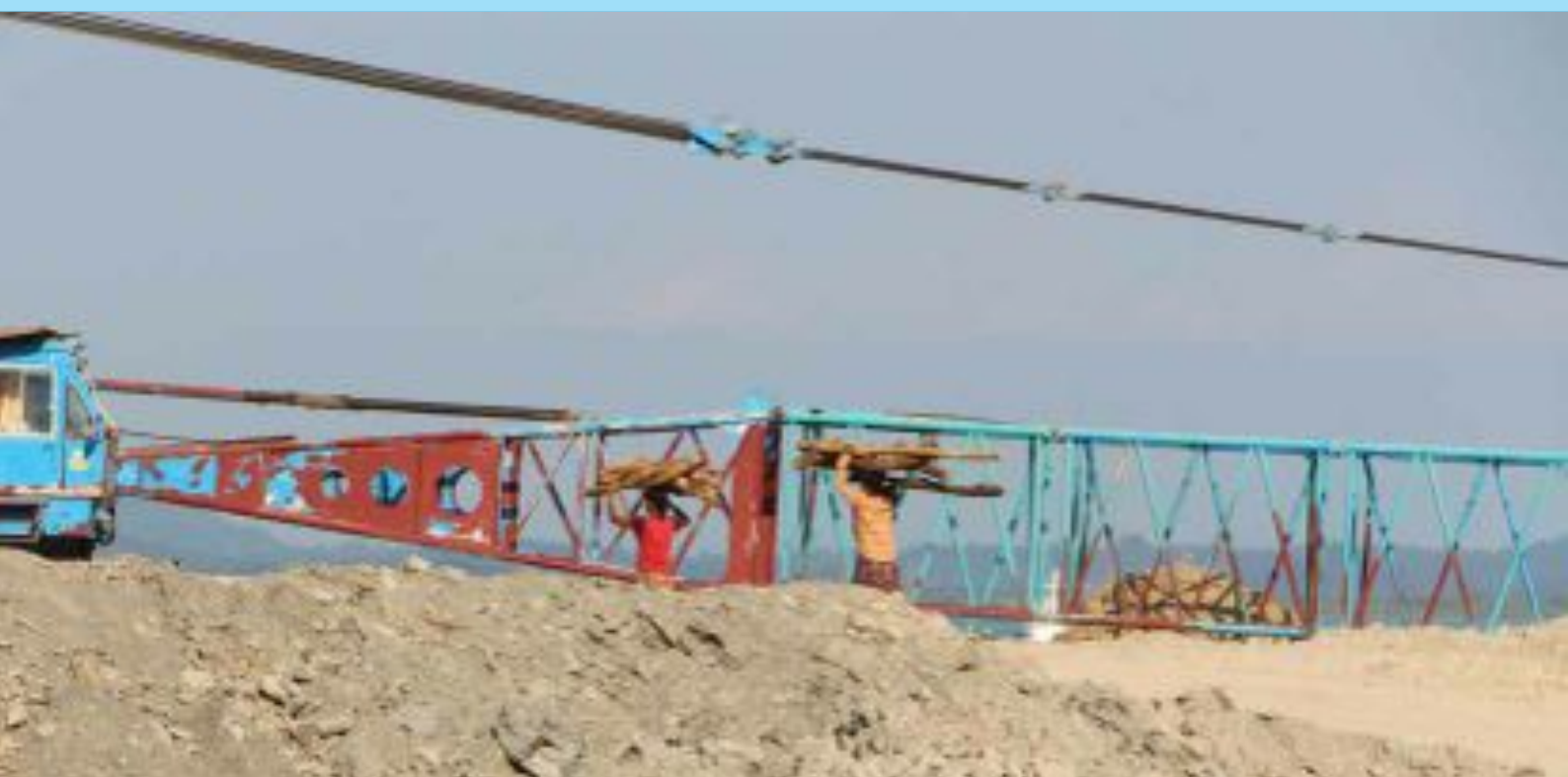
Below - Women carry firewood for cooking fuel at the deep sea port construction site, Maday Island.
