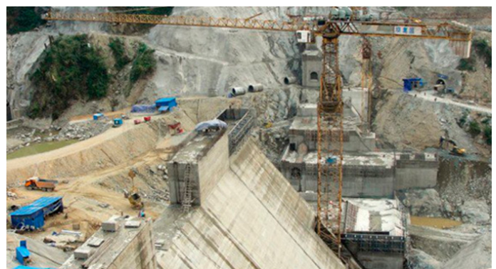
Construction of Myitsone Dam project in Kachin State. (Photo: Irrawaddy)
