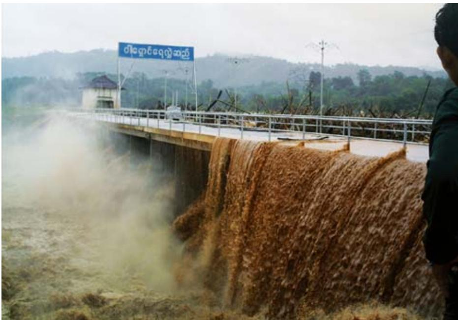
The Washawng Dam in Kachin State breaking in May 2006; the resulting flood completely destroyed the dam
